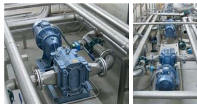
WATER TREATMENT PLANTS
