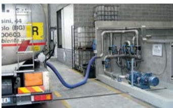
RECOVERY OILS PLANT
